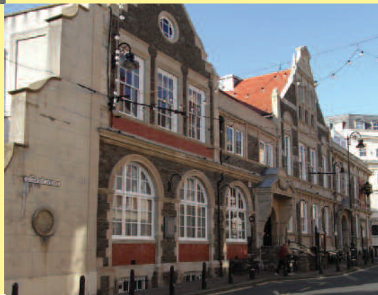
Town Hall following restoration work summer 2009
