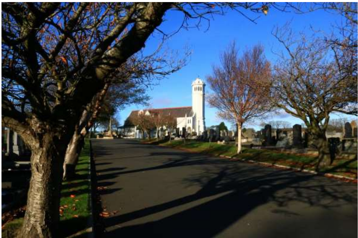
Douglas Crematorium across Glencrutchery Road serves the whole of the Isle of Man.
