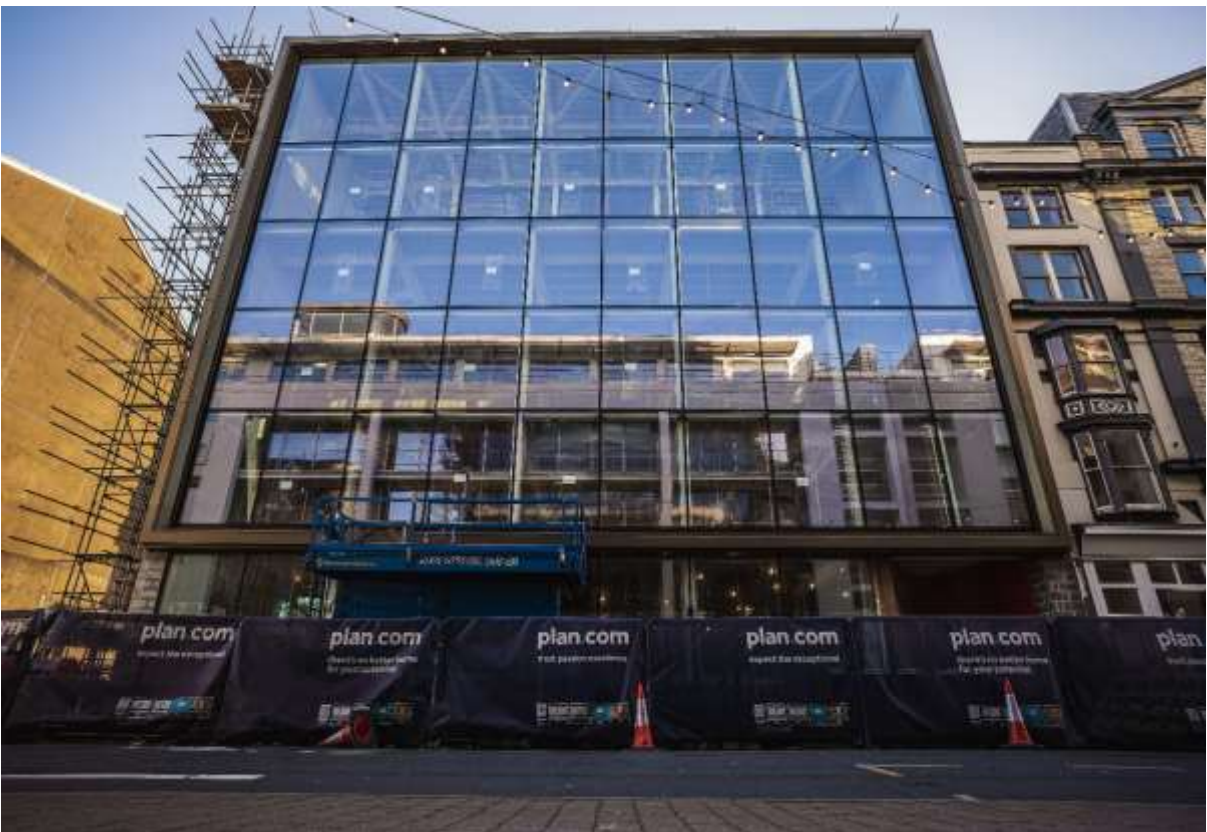
The new offices for Plan.com currently under construction on Victoria Street.
