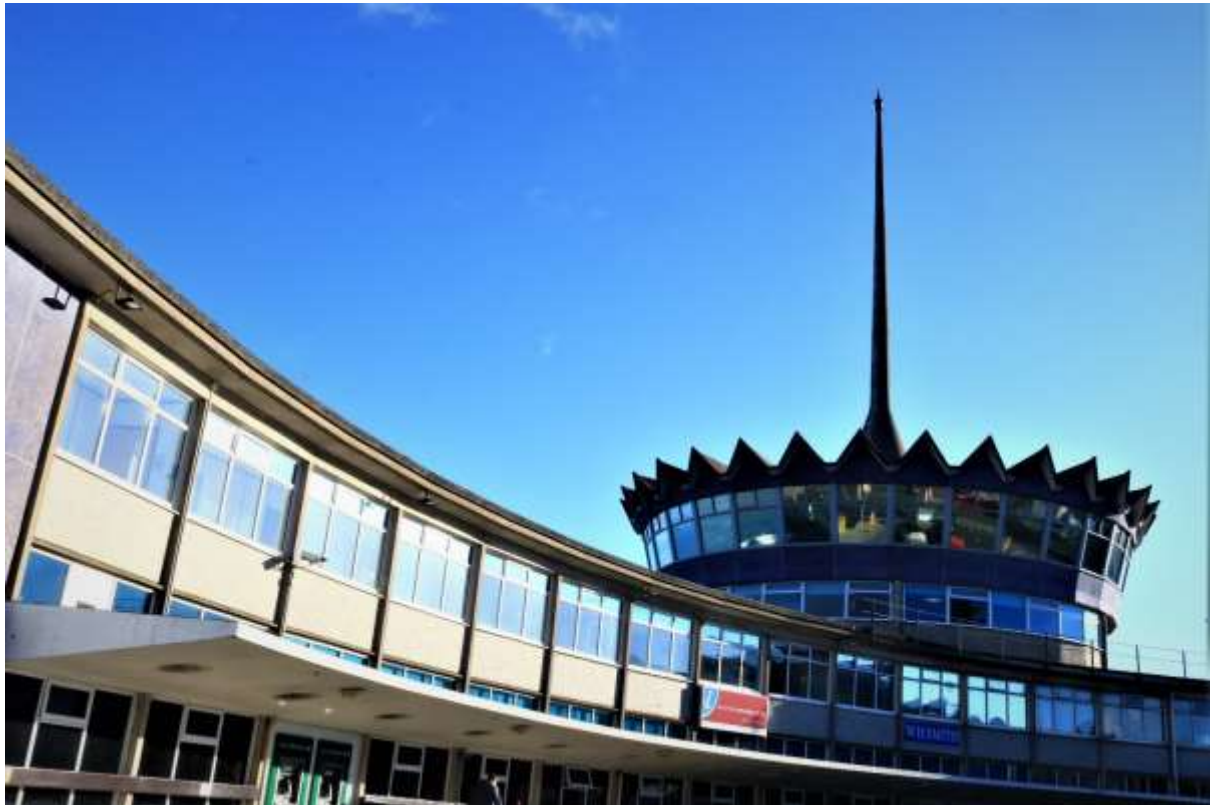
The iconic Sea Terminal building is the main landmark of Douglas Port with its crown shaped tower and three-legged footprint.
