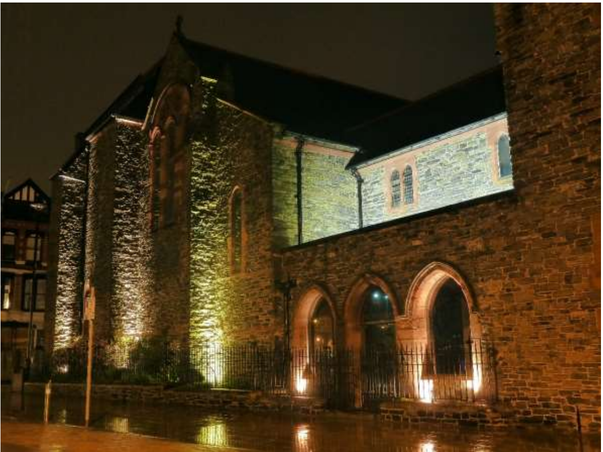
St Mathew's Church on North Quay is one of numerous buildings illuminated in the evening.
