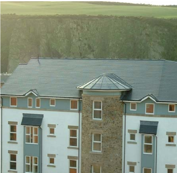
New Housing at Hanover House
